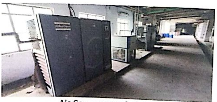
Air Compressor & Drier
